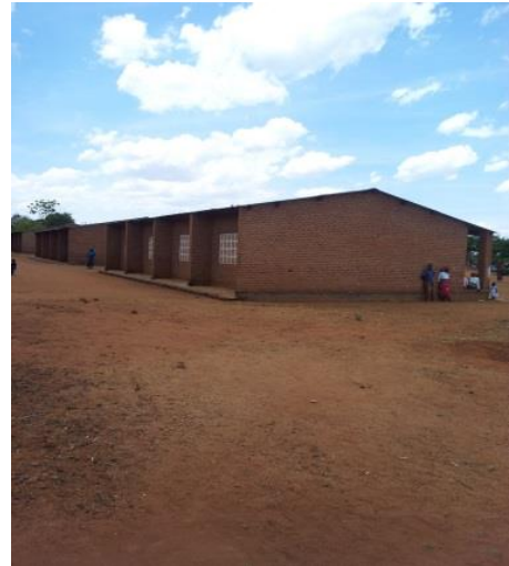
Figure 1 Nakanyanja Primary School. Photo credit: Harry Satumba
